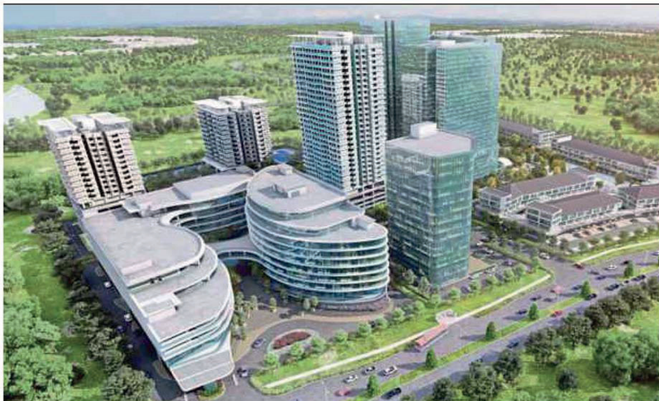
An artist's impression of Kerjaya Prospek Group Bhd's Edusphere @ Cyberjaya project. Public Investment Bank Bhd says the company continues to strengthen its portfolio by leveraging its core construction expertise while expanding its client base. PIC FROM KERJAYA PROSPEK'S WEBSITE
